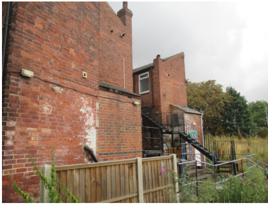
Wider view of 250 to 254 Derby Road
