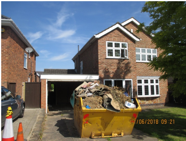
View of south east (front) elevation and boundary with no. 4
