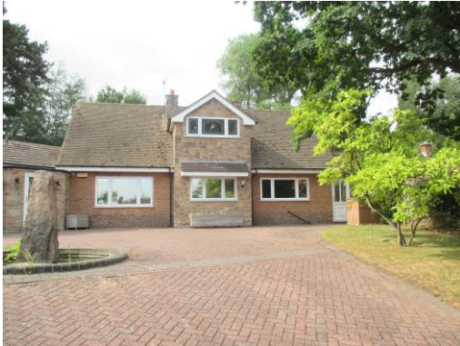
Extension prior to demolition
