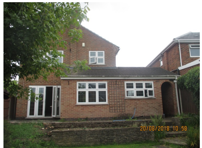
View of north west (rear) elevation
