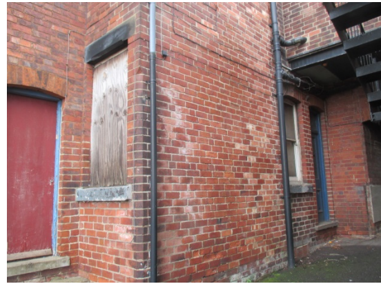
Detail of 248 Derby Road
